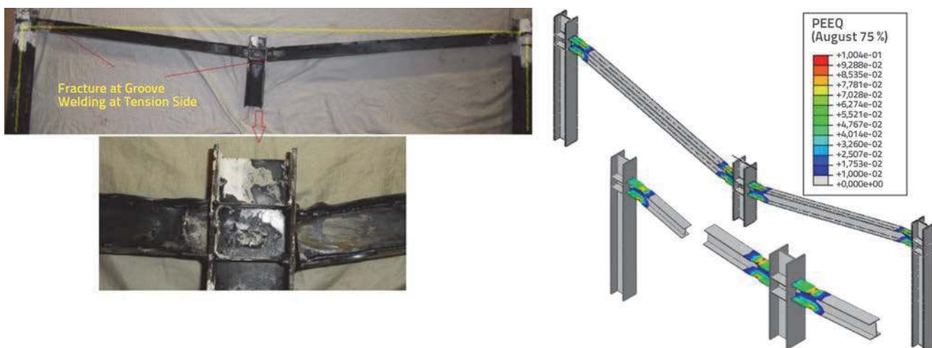
Figure 10. Specimen damage at the end of progressive collapse test and plastic equivalent strain distribution
